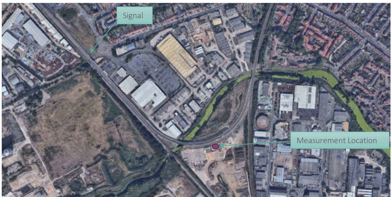
Figure 2: Curved Section of track at Hadleigh Road Industrial Estate, Ipswich – showing measurement location
